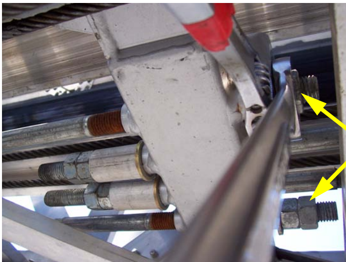
Cables Adjustment - Outer Jam Nut Retighten
